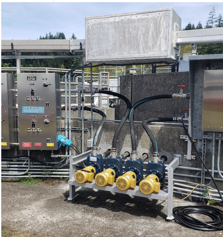
Newly installed Washington Shore LPS pumps (4/29/2021)
